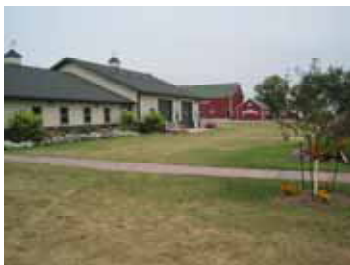
Read Memorial Bldg- 2012
