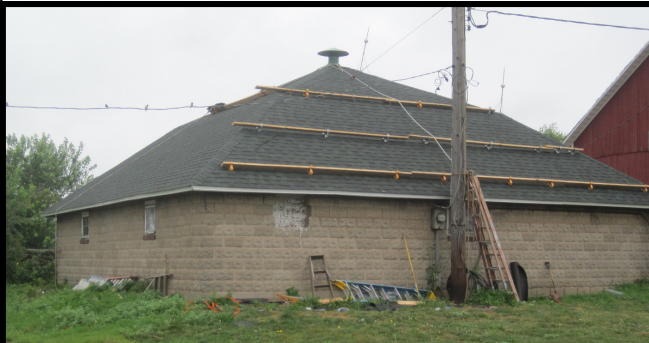
Shingling of Cold Storage Building
