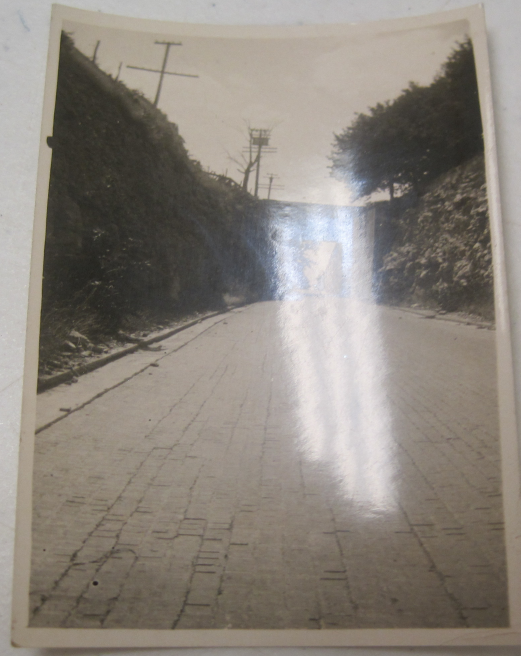
Bridge over Pekin Cut looking north. Work on the original cut was in 1917 with the bridge built later. Note the brick on the road.
